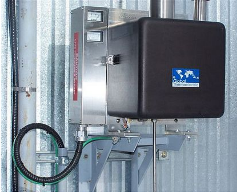
Figure 5. A thermoelectric generator. This has no moving parts so it lasts much longer than the generator shown in Fig. 4 (Gentherm Global Power Technologies).
