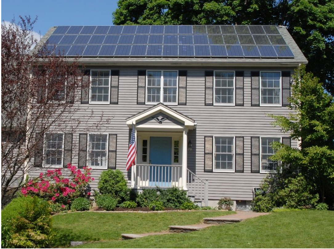
Figure 3. Solar panels produce 612 kWh/month in the upper Midwest (cleantechnica.com).
